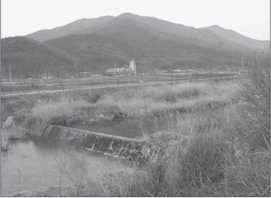
Figure 4. Ugok Diversion Weir at Togae Township, 2010
