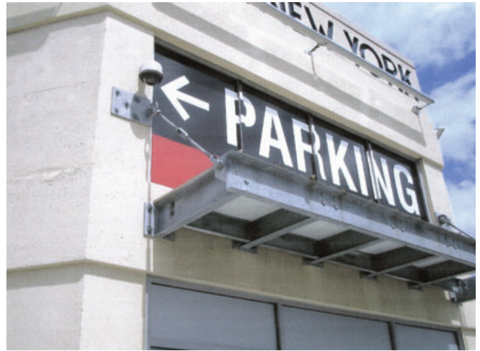
Figure 17. Building D looking north along River Avenue. The mid-20 th century Art Moderne façade was successfully restored and the structure was integrated with contemporary architecture of Gateway to its rear (Above). Modern fixtures attached to the front of Building D (metal awning and camera) continue the integration of old and new design styles (Below).
