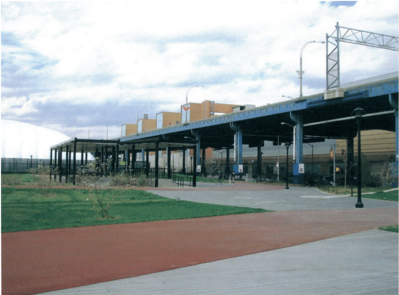
Figure 13: Mill Pond Park, looking northeast across Exterior Street (renamed Gateway Center Boulevard in 2009) and the elevated Major Deegan Expressway at Gateway. The large white bubble covers tennis courts. This park was built on the original 1900 landfill used for rail freight yards.
